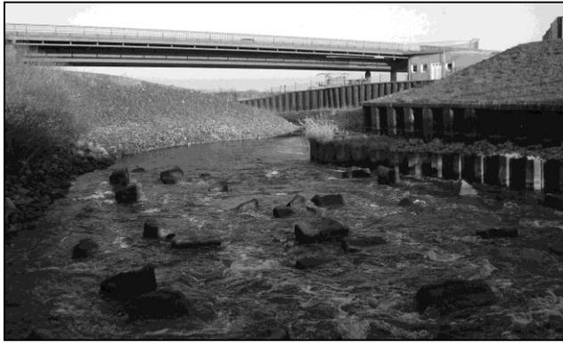
Figure 2. The natural-like bypass channel on the left bank of the Geesthacht weir
