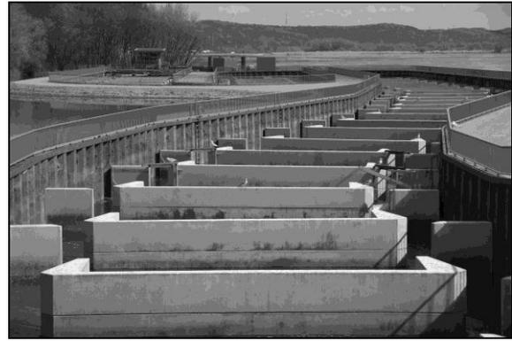
Figure 3. The double slot pass on the right bank of the Geesthacht weir
