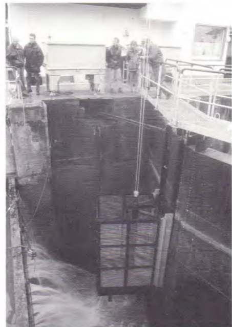
Abb. 3: Vor dem Schütz positionierte Fangreuse (abgedämmte Baugrube) Fig. 3: The upper gate of the ship-lock with the weir-basket (photo made during installation)
